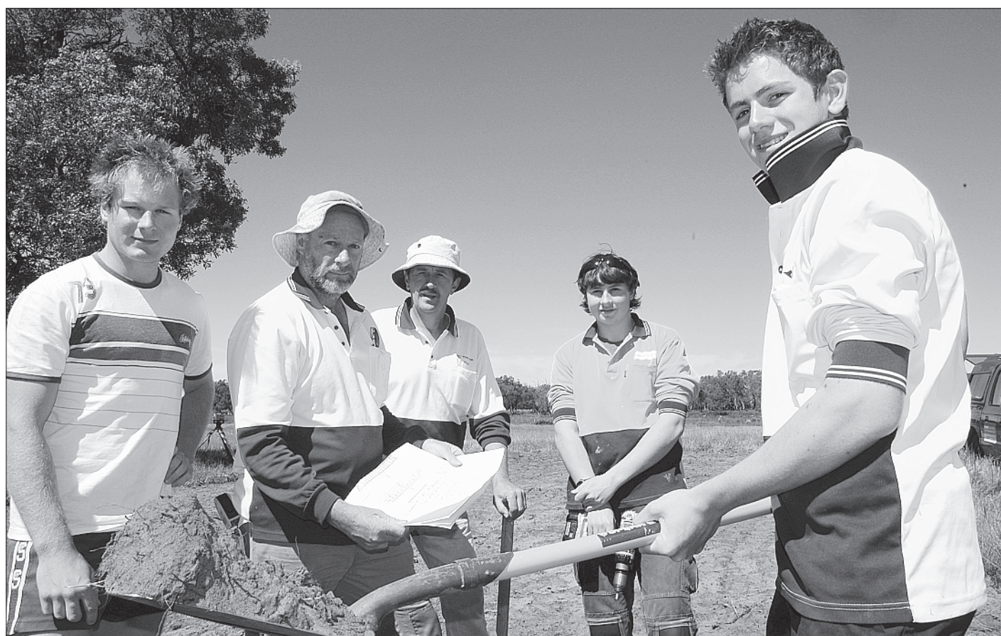
VALUABLE EXPERIENCE: Site manager Sam McPherson (left) stands with Building Trades trainers Mick Neu and Peter Larcombe as building students Cody Quin and Jaymie Dobie (front right) start work on the site office foundations. Picture: SANDRA MORELLO.
